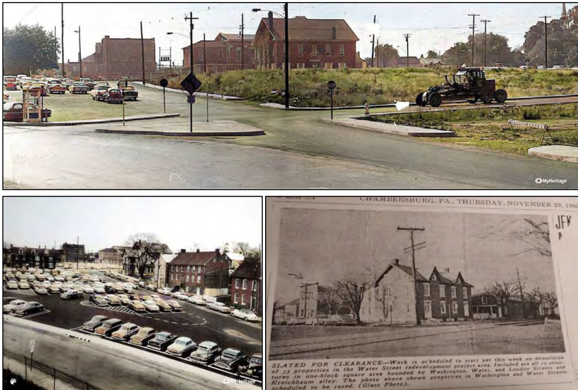
Figure 2-4: Water Street Redevelopment Project, Circa 1962
